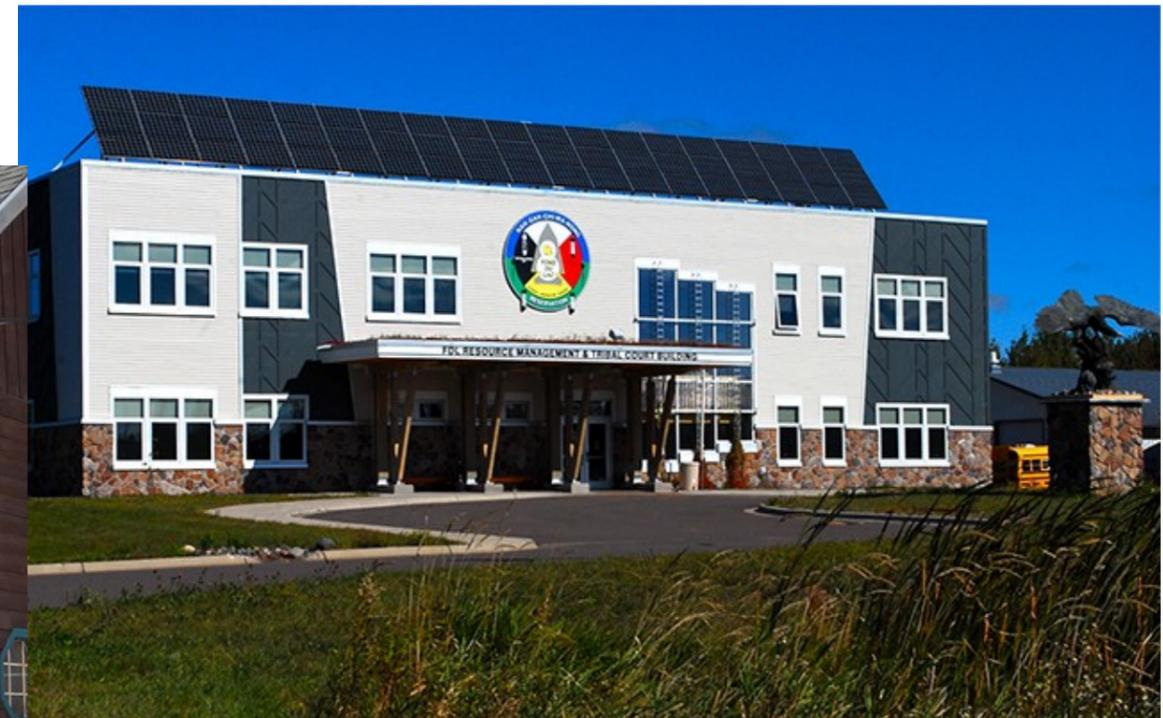
The Tribal Court/ Natural Resource Building is LEED certified which means it was built to use less energy than a standard building. Also to help reduce the carbon footprint of the reservation there is a 12 KW solar panel system on the roof of the building. These solar panels capture energy from the sun and turn it into electricity for the building.
